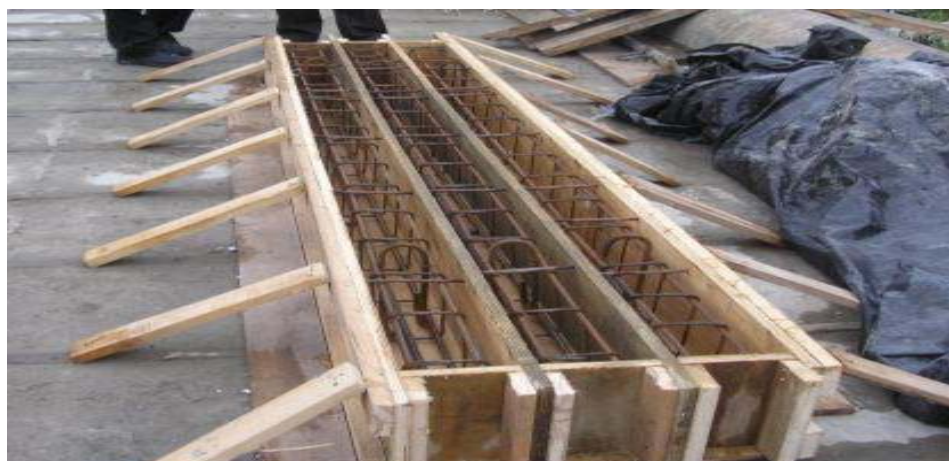
Figure 13. Moulds with placed reinforcement.
