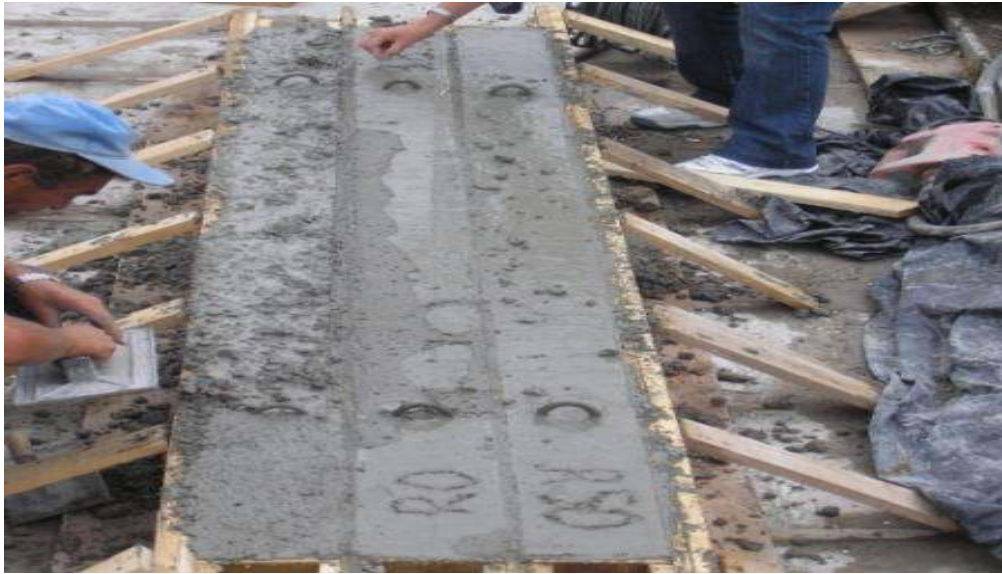
Figure 14. Finishing of the beams concrete surface.
